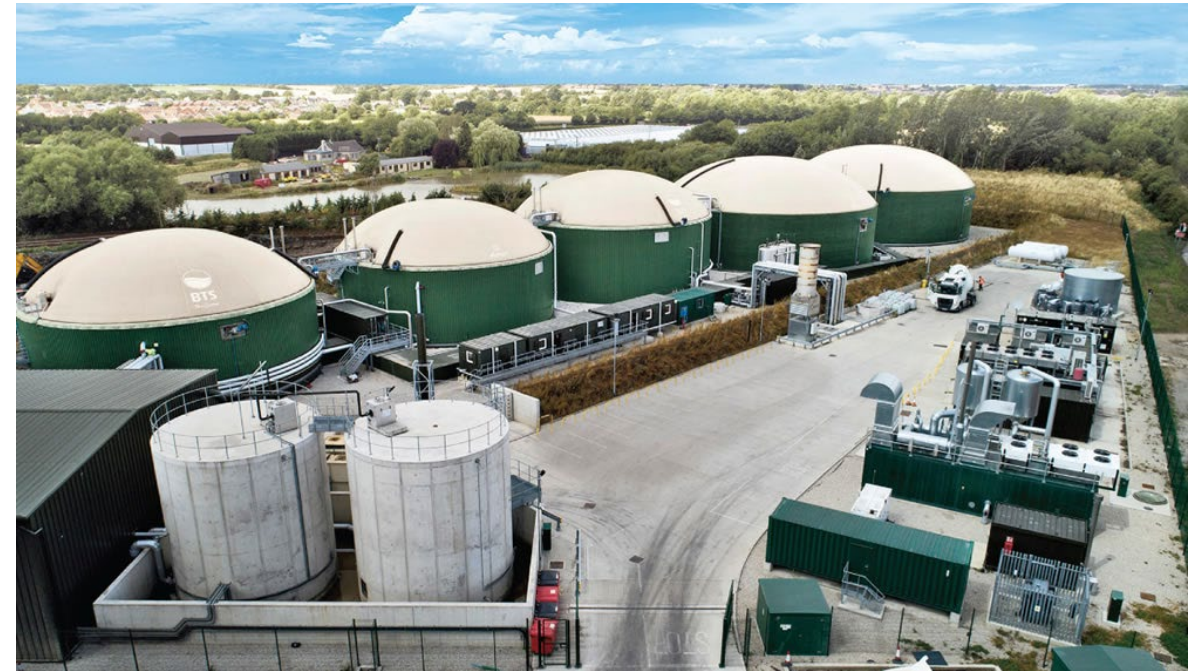
Figure 25: Anaerobic Digestion Facility
