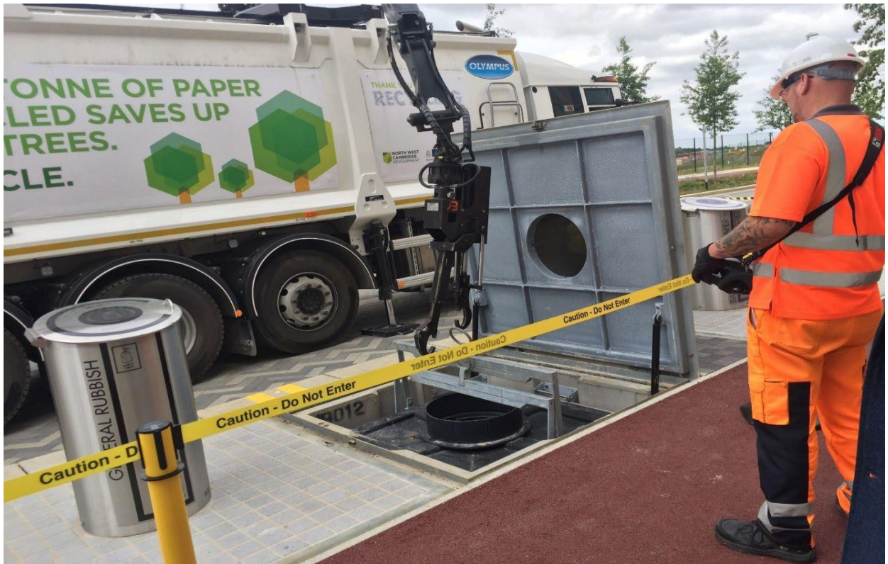
Fig 19 Underground bins hook-lift system in the ground
