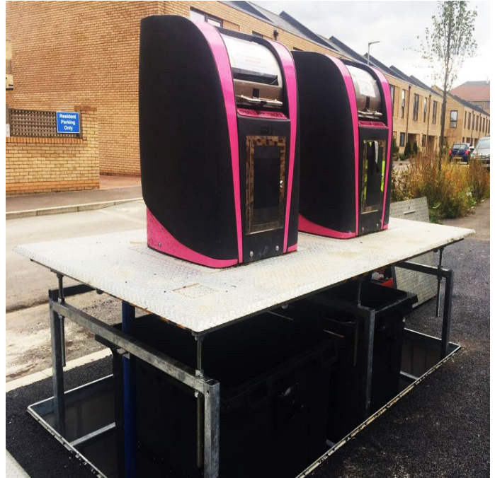
Fig 17 Double Hydraulic bring banks collecting mixed recycling collecting small electrical appliances
