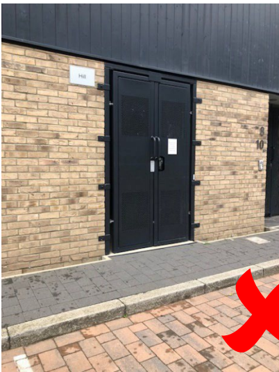
Fig 3 No drop kerb and pavement too narrow for 1100 litre bins
