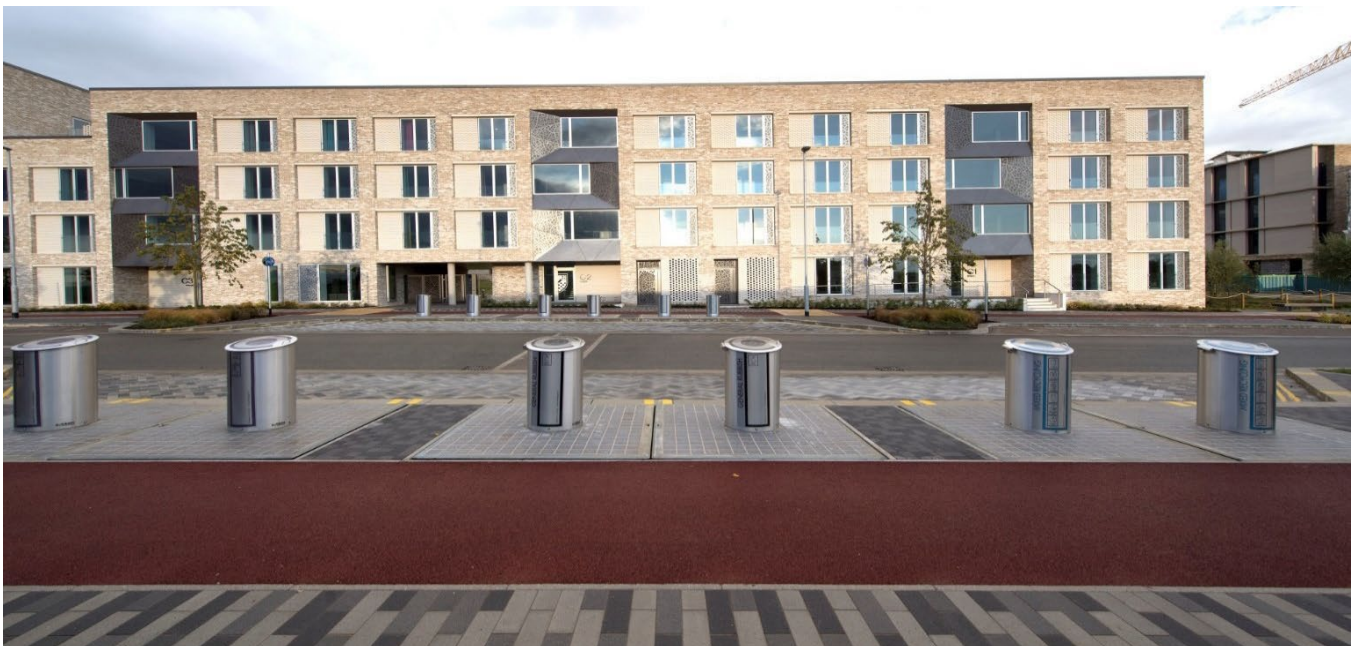
Fig 18 Underground bins hook-lift system streetscape
