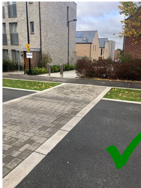
Fig 11 Swales are slatted to allow 1100 litre bins to be easily moved to roadside for collection
